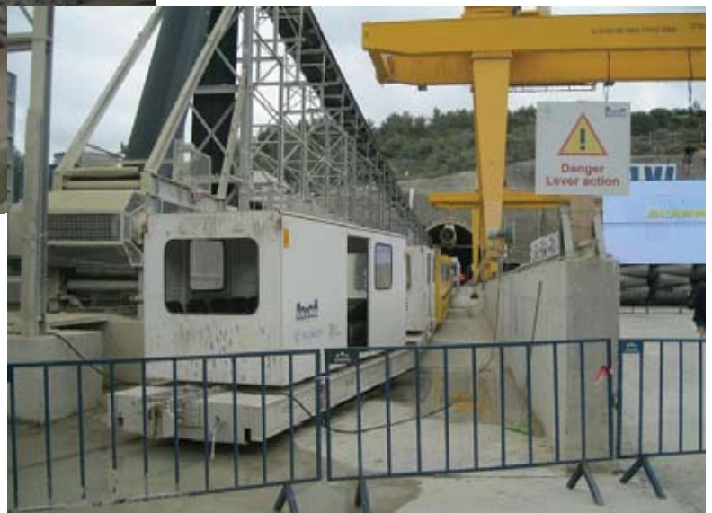
A works train, photographed "on dry land"
