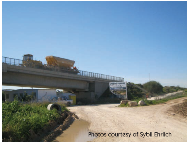
Ballasting Work on high-speed line 04.02.2016
