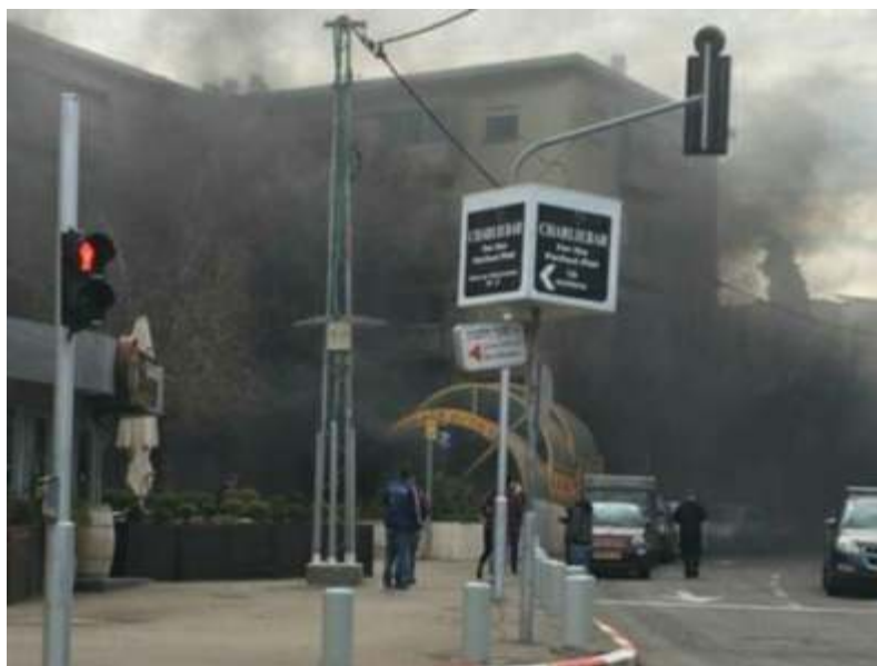
The heavy smoke coming out from the entrance to the Mother's Garden station on the Carmel (the building with the yellow roof).
