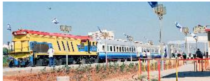
• Picture 10: The first air-conditioned train at Herzliyya's refurbished station 23.10.1989
