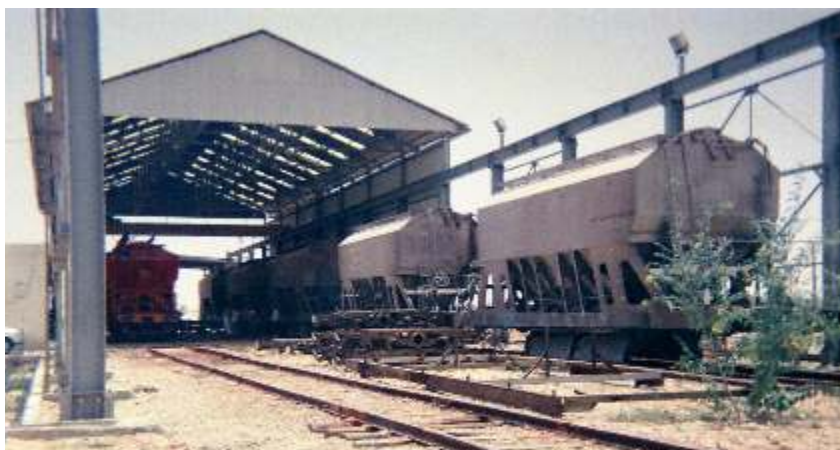
• BREL wagons undergoing maintenance at the wagon repair workshop at Beer Sheva in Summer 1982. At that time the facility was sub-contracted by ISR to Kadmany Metal Works. (photo: Harel Even)
