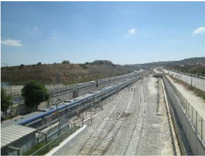
• The newly-expanded Paatei Modiin Station (Photos Marion) in August 2021. Electrification has not yet commenced. (Photo courtesy of Steve Sattler)
