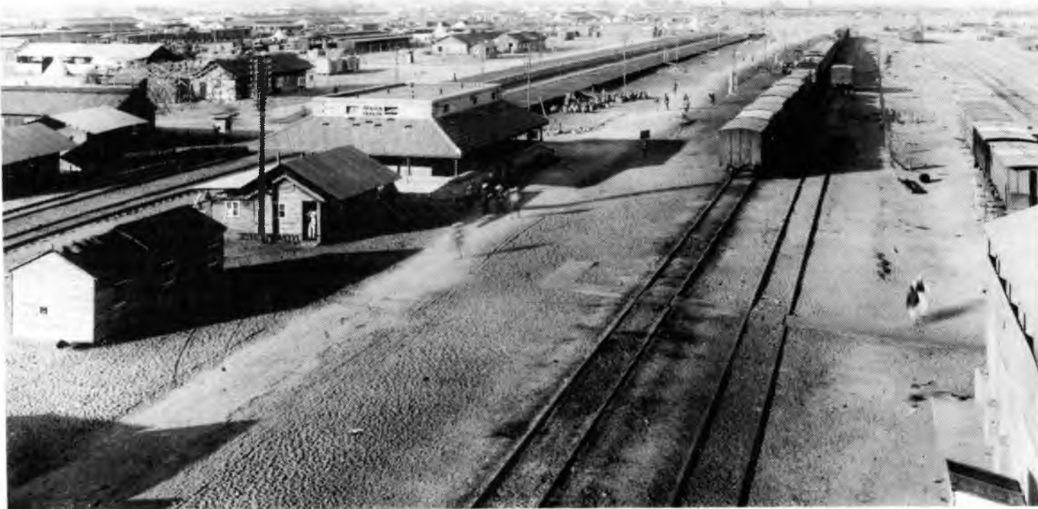
21:13. : Kantara East Station Buildings - a glimpse of the vast array of tracks and facilities laid out here to service the British campaign across Sinai and into Palestine. No exact date - probably 1918. Note trees in the distance marking the line of the Canal; double-skinned roof over one of the wooden huts (to reduce the temperature inside); and several Egyptian 6-wheel coaches parked on an isolated track to Right, used as offices.
