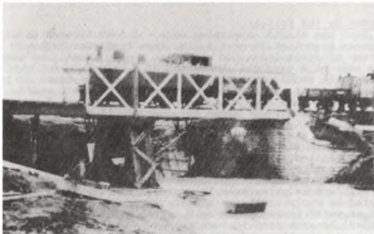
An indistinct photo of what is believed to be "the big bridge at Sedjed" over the Wadi Surar. It appears to have been taken in the winter of 1917-18, and there is evidence of a washout with temporary repairs being made. The loco is a La Meuse 2-6-2T which helps to date this view as being sometime fairly soon after the British captured 'Junction Station' in November 1917 but before the line to Jerusalem was standard-gauged the following spring. (This section converted in March 1918) (Photo: Paul Cotterell Collection).
