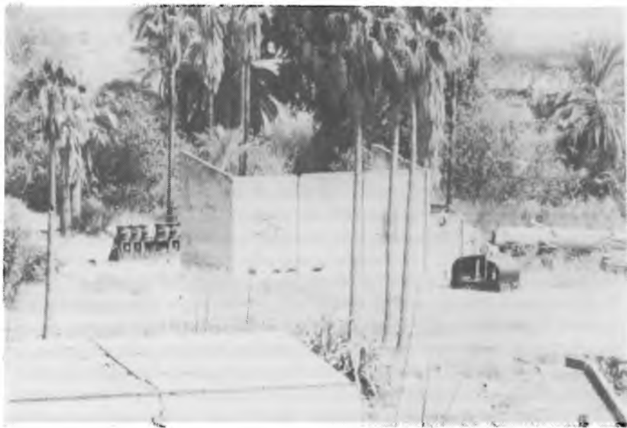
1. Looking across the power station site from the observation point on the Israeli side of the River Jordan. A corner of the turbine house can be seen at lower left. At right is the body of the Hibberd petrol locomotive. 5/10/94.
