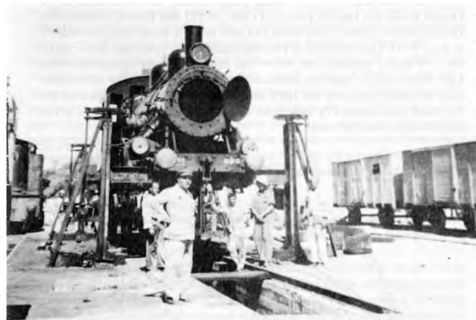
31:21 Kantara East: Baldwin 4-6-0 NO. 886 on the lifting jacks. April 1948. A steam crane with vertical boiler is just visible on left.
