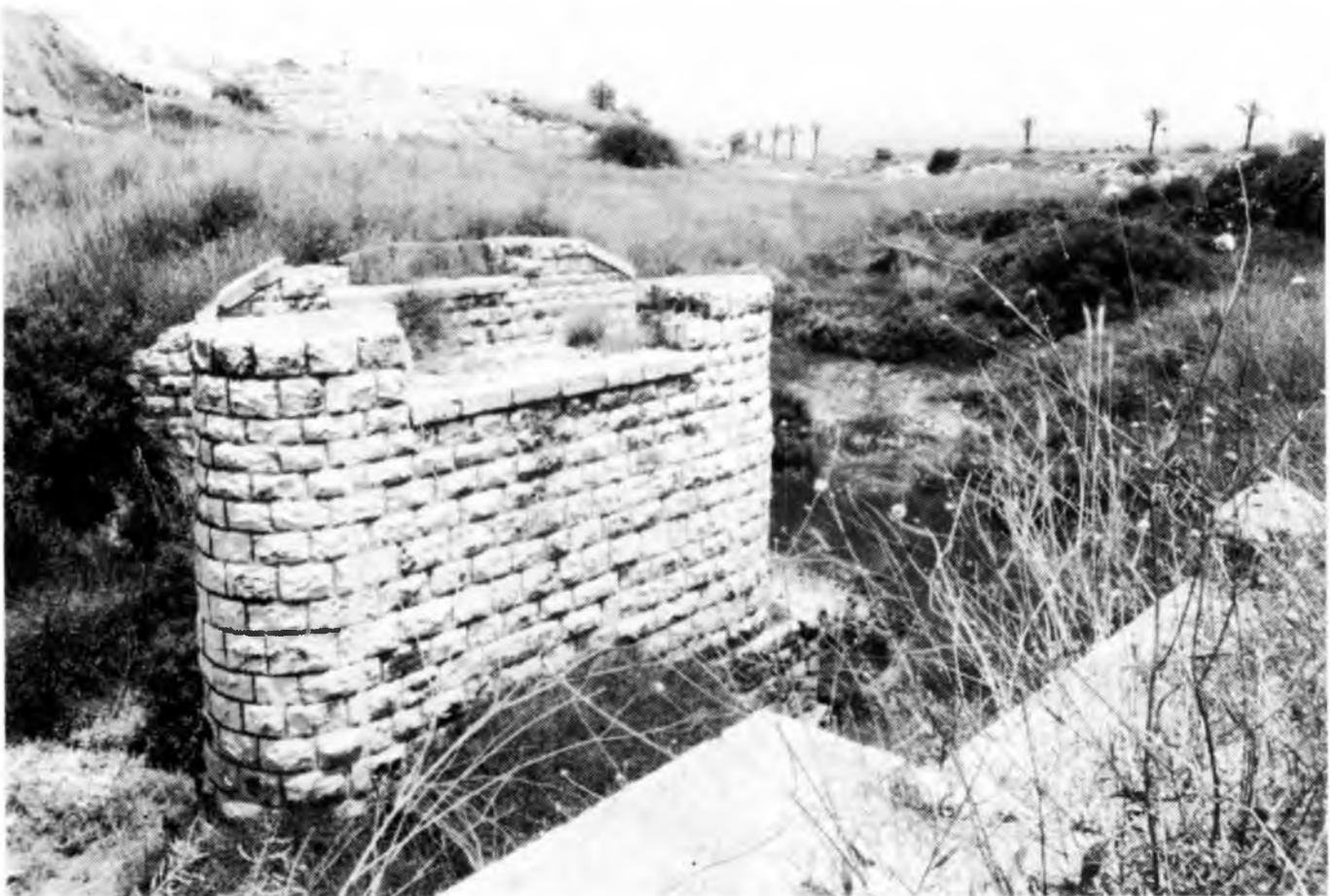
Remains of the bridge over Nahal Beit Arif, looking east.
