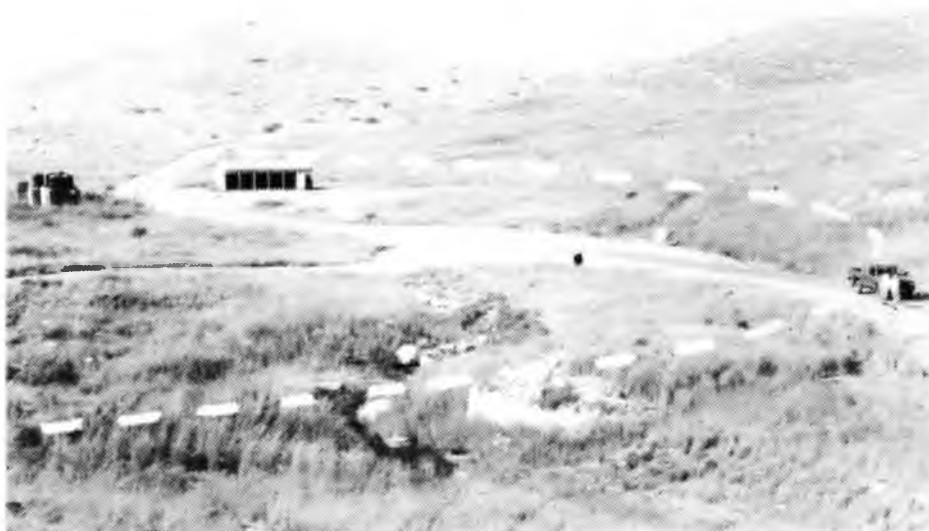
Photo 3: The ruined bridge across the side stream at the presumed site of Qum ez Zawan siding. David Menachem's 4x4 truck stands on the narrow gauge formation which curved round behind the army firing range and disappeared in the patrol road. Approximate route is indicated by the dotted line. 26/9/97.
