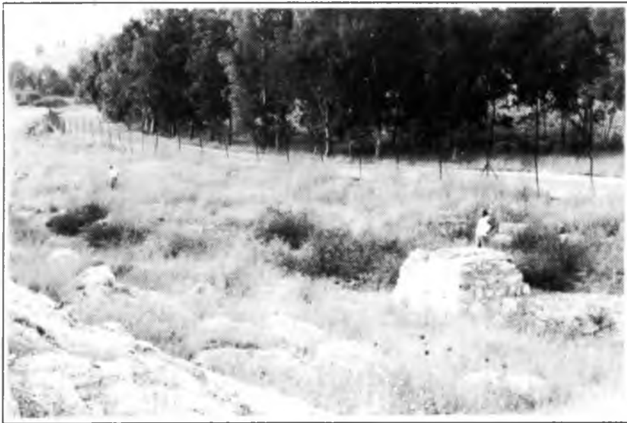
Photo 1: Remnant of a bridge abutment over Wadi Bet Arif, looking north towards the rubbish tip. The narrow gauge line seems to have crossed the road and continued on more or less parallel to the row of trees. 26/9/97
