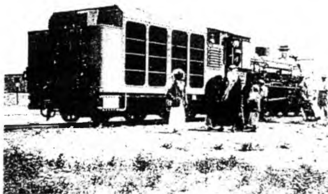
Iraqi State Railways class HG locomotive no. 127 with a condensing tender. Photo courtesy of Iraqi State Railways.
