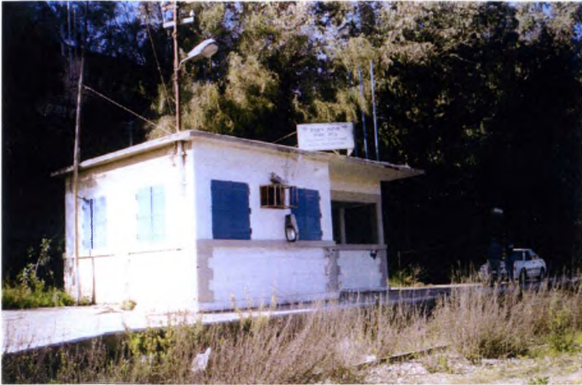
Beit Shmesh Station as it will never be again. The Upper photo shows the signal box and station building as it was in February 2002, the Lower photo (facing towards Jerusalem) shows the station tracks totally overgrown. (Photos: Sybil Ebrlich).
