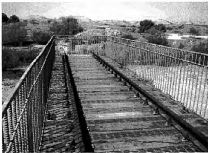
3. Looking west along the new replica trestle bridge over part of Wadi Shellal in March 2004. The original track curved slightly to the right on the other side of the Wadi and then left into a short cutting which was dug by Sikh Pioneers of the British Army (see contemporary photos in AWM Photo Database). (Photo: Erez Shalev.)
