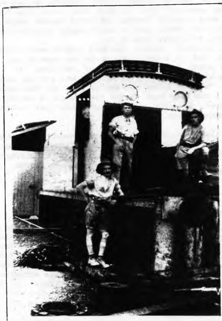
Manning-Wardle petrol loco. for armoured train - under repair at Kantara Workshops. It appears the engine has been removed from the frames.
