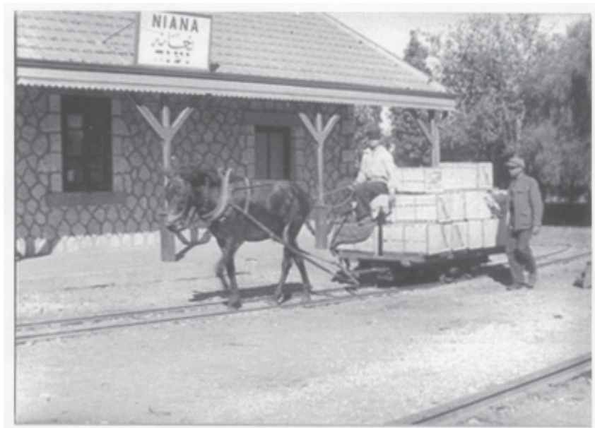
One horsepower locomotion for one loaded flat wagon of citrus fruit arriving at Niana station from Gan Hadar. The standard guage main line of PR is glimpsed at bottom of picture.
